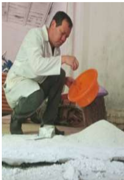
1-picture. The process of sprinkling quenched lime
