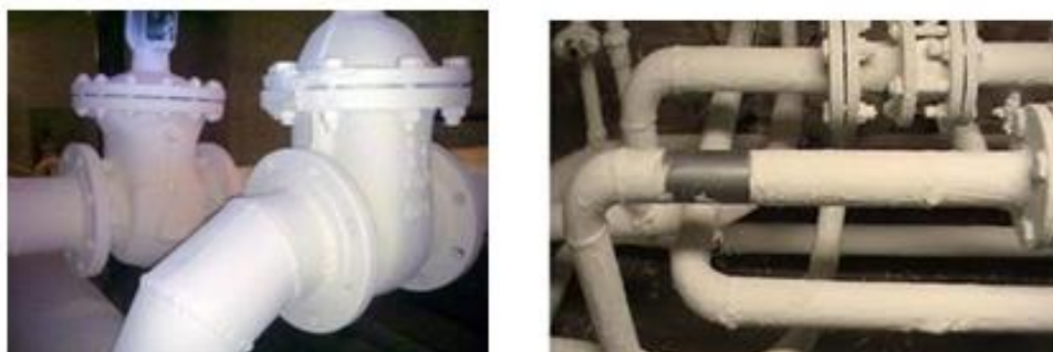
Picture. 2 Coating on surfaces that are considered complex
